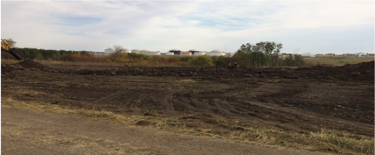
West side of Pipestone Creek Clearing for Laydown area.
